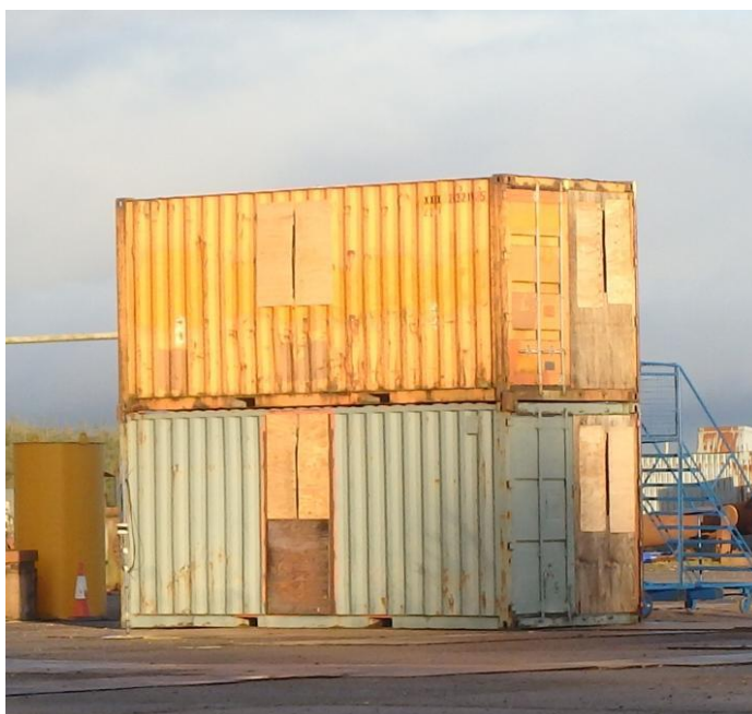
Figure 43 Containers used as a model two-storey enclosure in Cleaver et al. (2016). Openings can be observed on the front and sides of both floors (© IChemE copyright 2016)
